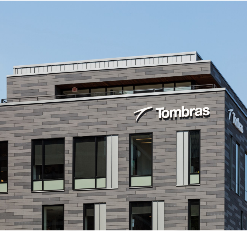
View of the penthouse area atop the Tombras Group Headquarters
